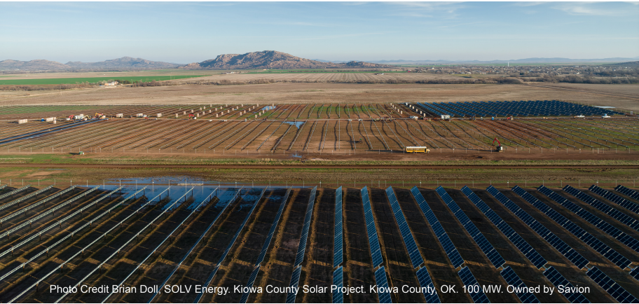
Photo Credit Brian Doll, SOLV Energy. Kiowa County Solar Project. Kiowa County, OK. 100 MW. Owned by Savion
